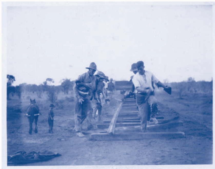
Men laying the last section of the line between Wire Creek and Alice Springs between 1927 and 1929. (Photo from the Joe Davis Collection, courtesy NT Archives Service)
