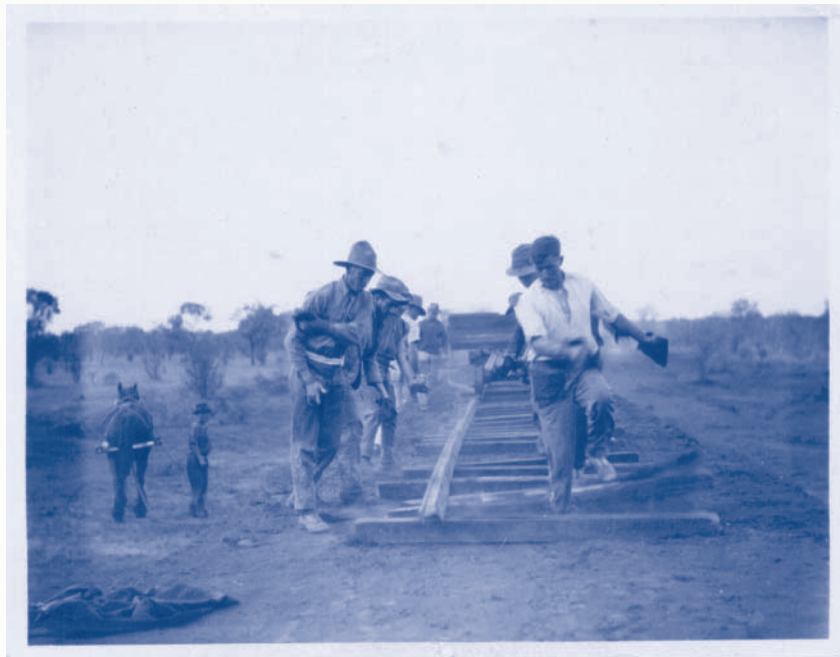
Men laying the last section of the line between Wire Creek and Alice Springs between 1927 and 1929. (Photo from the Joe Davis Collection, courtesy NT Archives Service)
